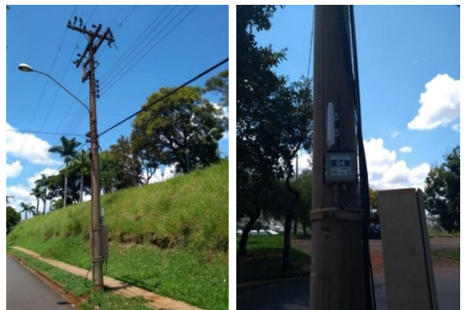
Figure 12. Installation of PLC system (coupler/ transceiver/radio) on substation side.
