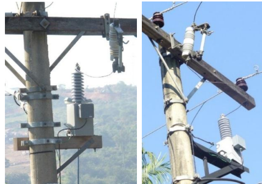
Figure 5. Details of coupler installation on the power line structure.
