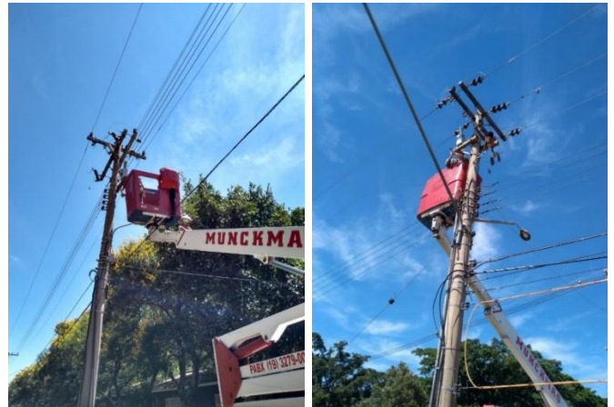
Figure 11. Installation of PLC system (coupler/ transceiver/SEL relay) on equipment side.
