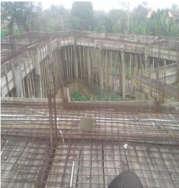
Figure 4. Picture of Steel Reinforcement of School of Post Graduate, FUTA
