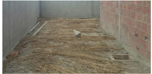
Figure 3. Construction Waste. Source: Author (2015).
