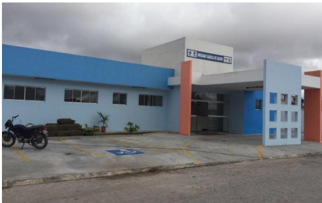
Figure 1. Construction completed. Source: Author (2015).
