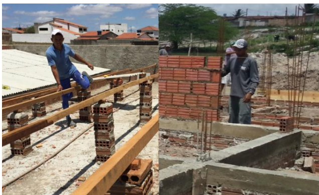
Figure 7. Construction Workers. Source: Author (2015).
