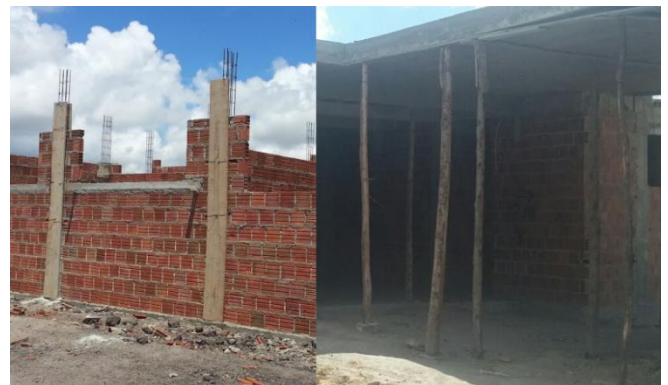
Figure 8. Shapes and shoring. Source: Author (2015).
