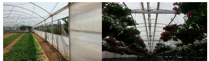
Figure 2. Ventilation on wall and roof in the greenhouses
