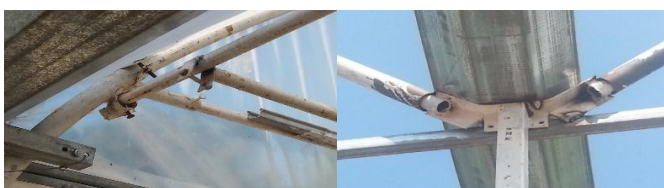
Figure 1. Joining type of metal elements (screw, welding)
