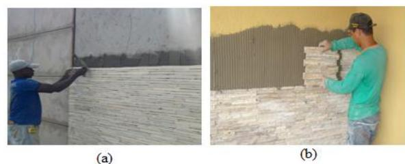
Figure 2. Application of stone (a) filleted, (b) ready stone plate.
