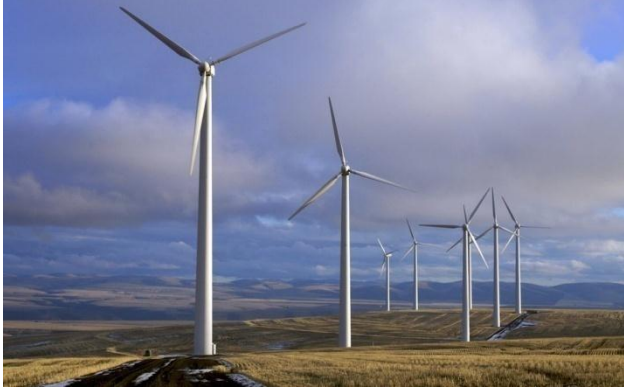
Figure 2. 199 KW wind turbine
