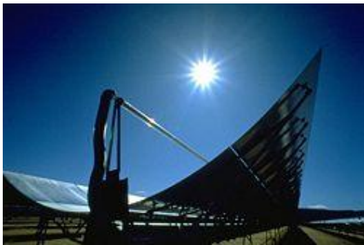
Figure 3. Linear 259 KW parabolic power plant
