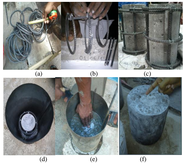
Figure 3. Preparation of Specimens for concrete confinement (a) Check for diameter of ties; (b)caging; (c) Encasement of plain concrete, (d) Plain concrete-reinforcement arrangement placement; (e) Pouring of concrete mix ( f'_c=4 ksi); (f) Resulting Strengthened Cylinder
