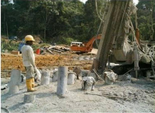
Figure 10. Slightly inclined micro- piles [6]
