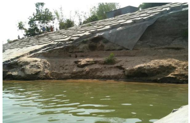
Fig. 2: Jamuna river bank after failure of a bank protection structure.
